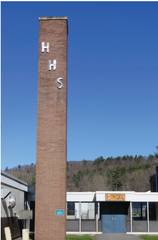
New school lettering on chimney.
