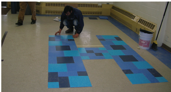
Installers working on new lobby tile floor design.
